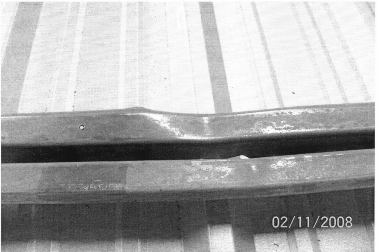
8X2.5ZEE 12 GA. TEST #1 FAILURE
